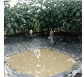
Plate 15. Farmer (Mikhail Abraham) working on rainwater harvesting at Katena Andi (Arbrakete) near Kuni in 15 m x 15 m x 2 m pond (N 9°02'40.8" latitude, E 40°54'39.4" longitude, 2299 m altitude). The programme is sponsored by the Ethiopian Government. The bottom of the pond is covered with plastic to minimize seepage loss and side is planted with castor to minimize evaporation by shadowing.
