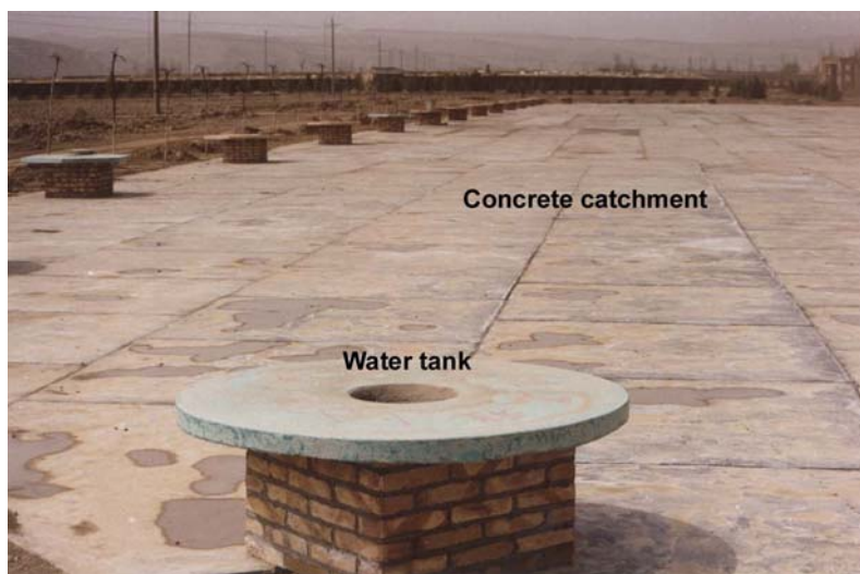
Figure 1. Rainwater storage tanks with concrete catchment for greenhouse irrigation, Dingxi County, Gansu Province.
