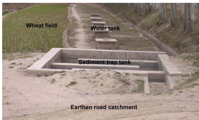
Figure 2. Water storage tanks distributed in the wheat field for supplemental irrigation.
